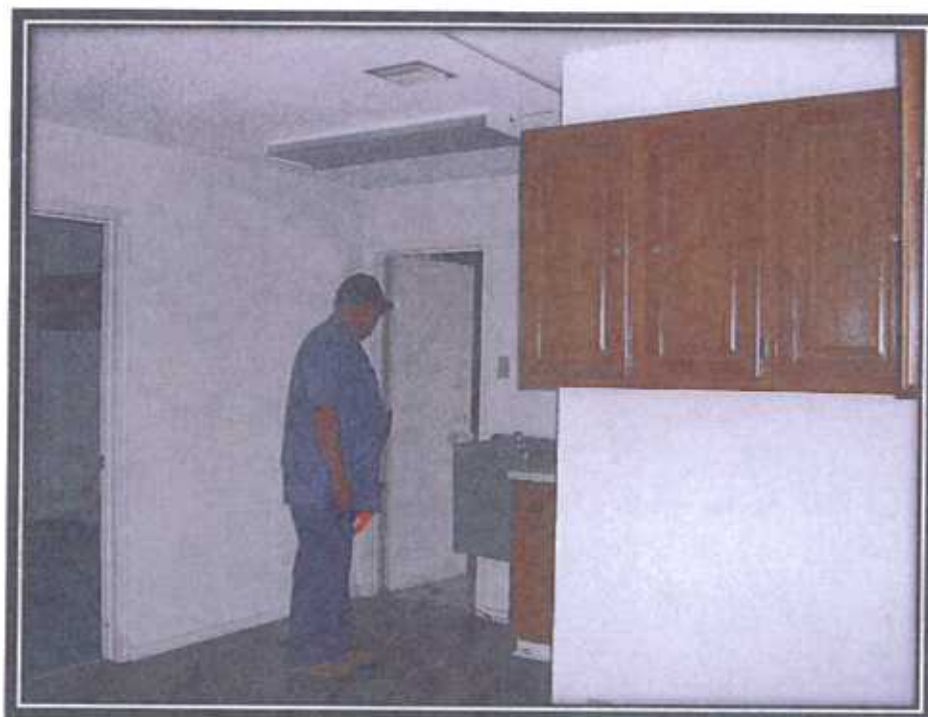
Interior view of the office building.
