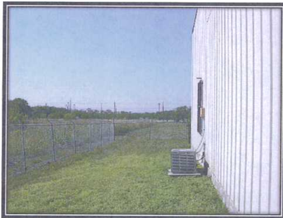
View of the east side of the metal warehouse looking south.
