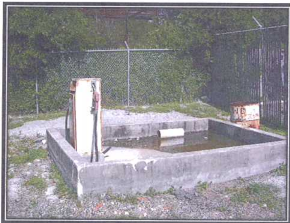
View of the second fuel tank looking west.
