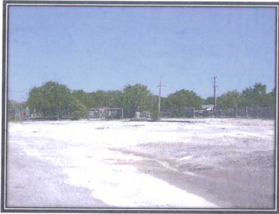
View of the yard area looking northwest.
