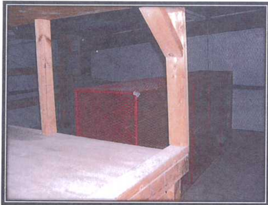
View of the second floor loft located in the northeast metal warehouse building.
