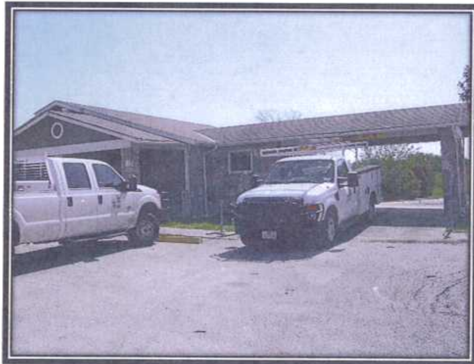
View of the drive-thru teller window located on the south side of the building.
