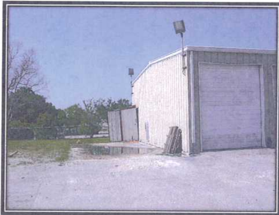
View of the east side of the larger metal warehouse building (containing 3,040 square feet).
