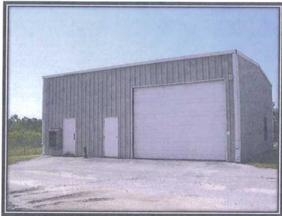
View of the metal warehouse building located along the northeastern portion of the site.
