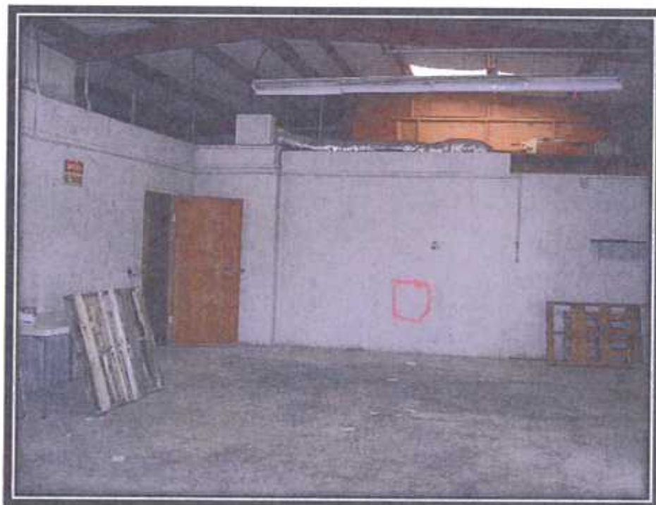
Interior view of the warehouse area.
